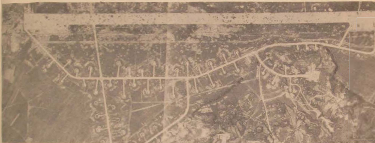
Taechon airfield, with a 6500-foot by 200-foot concrete runway built in October 1951, is systematically bombed and just as systematically repaired. This photograph was taken a day or two after a heavy bombing had shattered the runway. Repairs are already under way at both ends of the runway and will rapidly work toward the middle.
